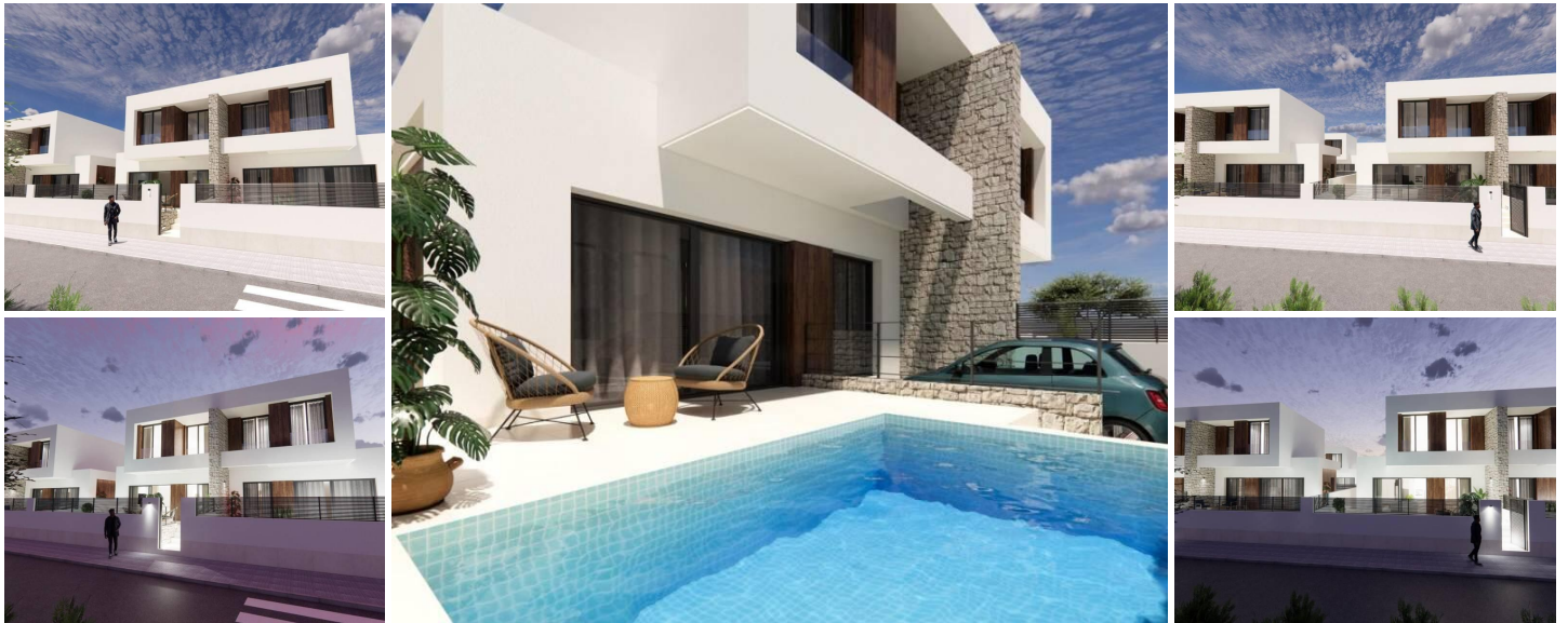
New Build Semi detached villas in Dolores
