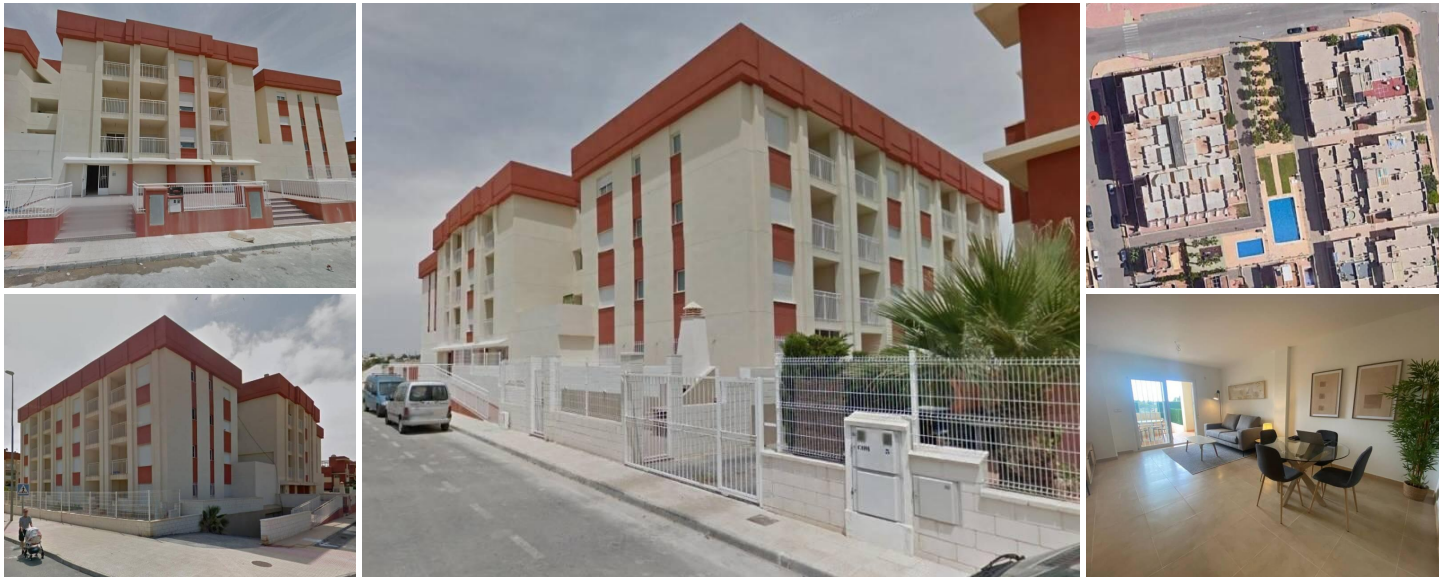
Regenerated Residential Complex in Lomas de Cabo Roig – Renovated Apartments
