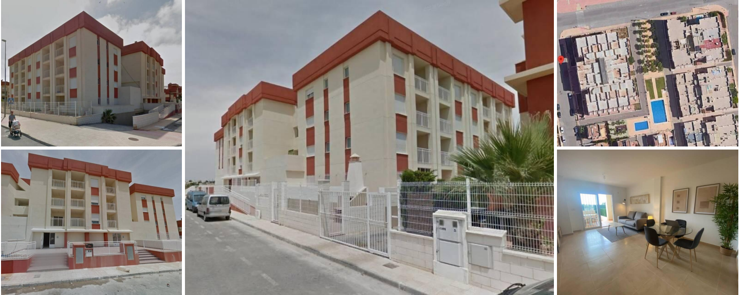
Regenerated Residential Complex in Lomas de Cabo Roig – Renovated Apartments
