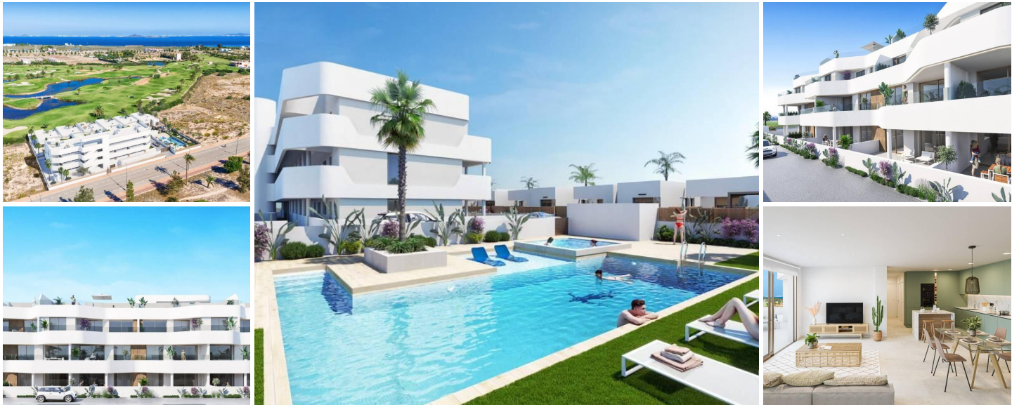
New Build Residential complex in Los Alcazares
