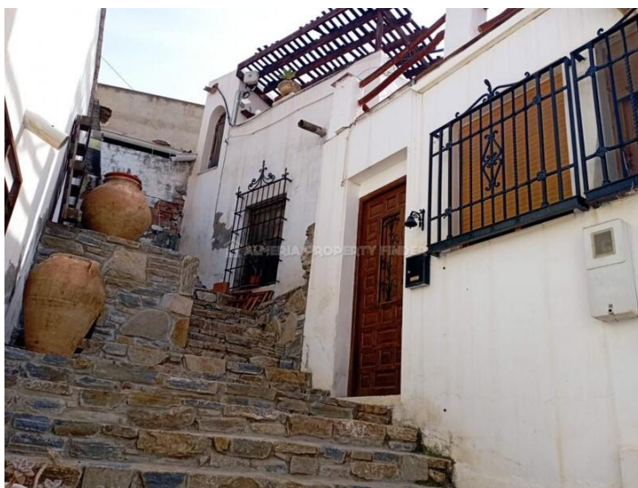
Casa Eva - A village house in the Sufli area. (Renovated)
