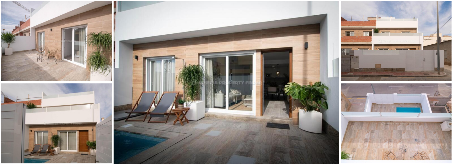
Aire Limpio III - T2 - A town house in the Avileses area. (Newly Built)
