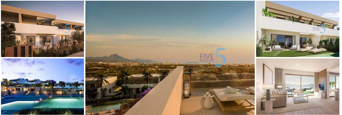
NEW BUILT CHALETS IN VISTAHERMOSA (ALICANTE)
