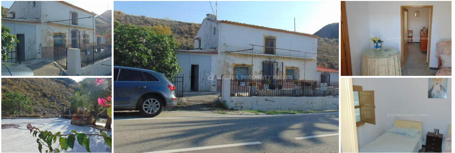
Cortijo Paco - A country house in the Arboleas area. (For Renovation)
