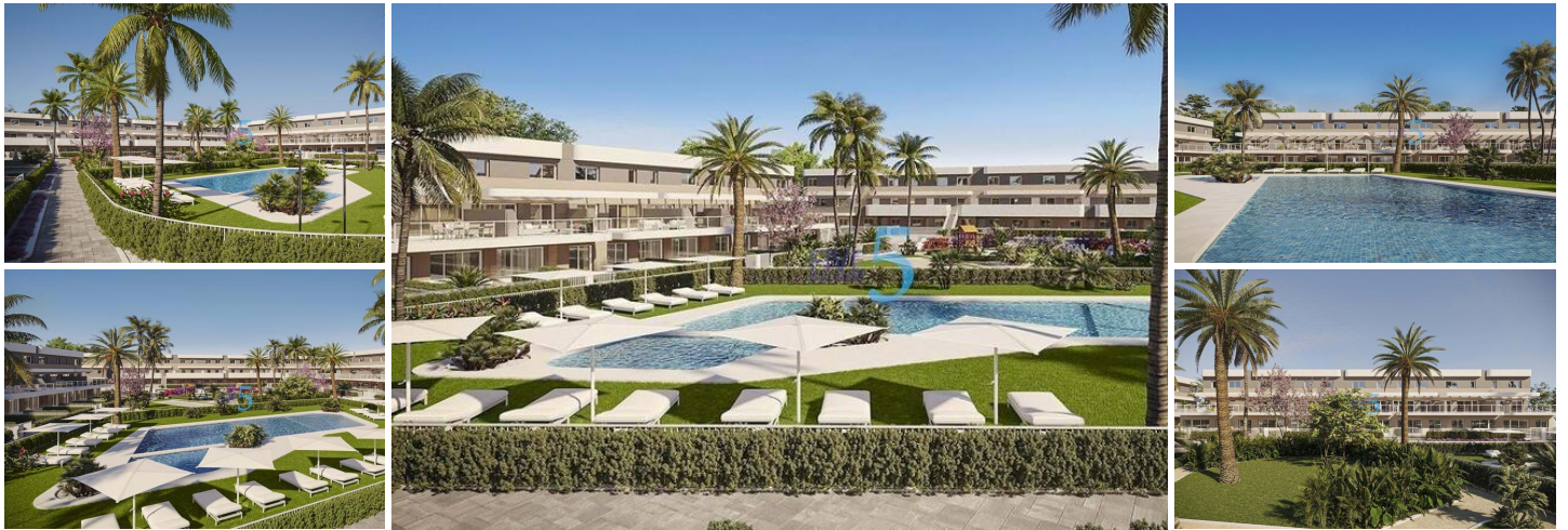
NEW BUILD RESIDENTIAL COMPLEX IN ALENDA GOLF, ALICANTE
