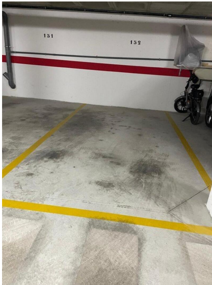
underground parking at Valentino golf block 4 in Villamartin
