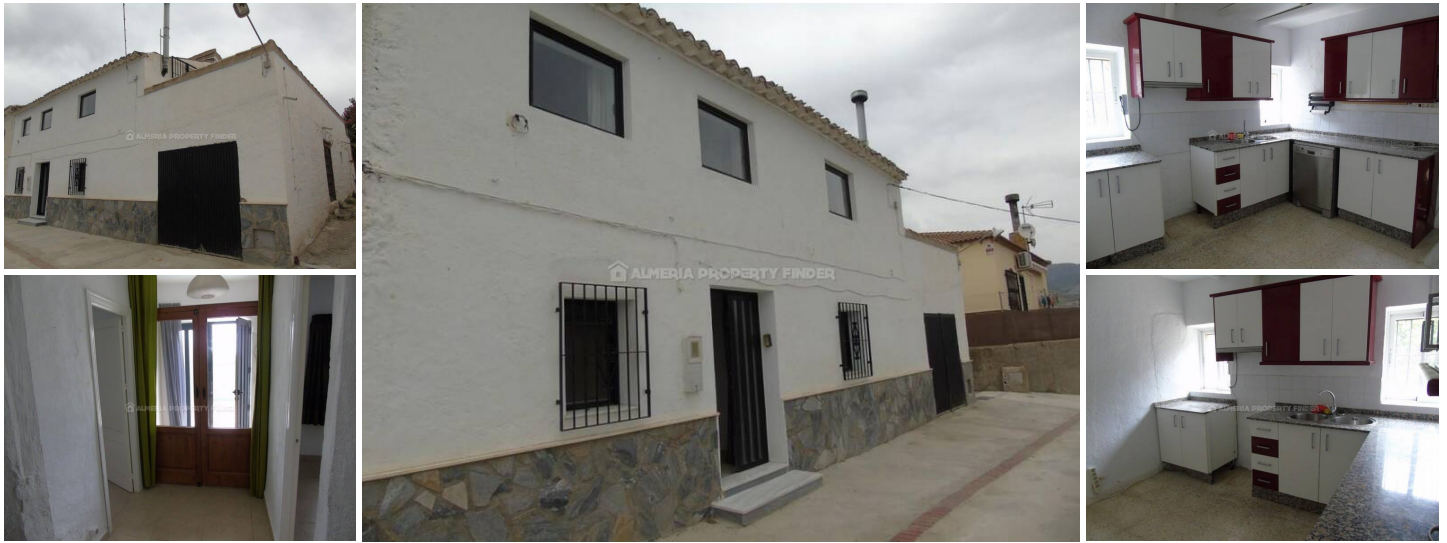
Casa Jirafa - A village house in the Cela area. (Renovated)
