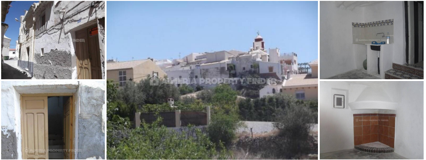
Casa Marion - A village house in the Somontin area. (Partially Reformed)
