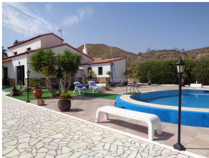
Casa Sanchez - A country house in the Arboleas area. (Renovated)
