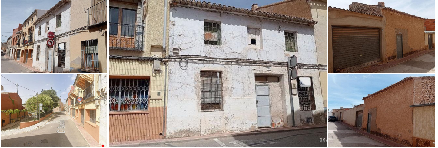
Huge Restoration Project in Caudete. More info to come
