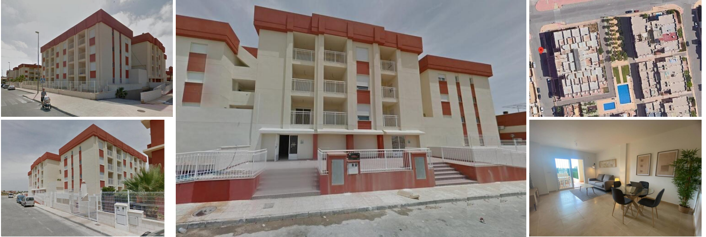
Regenerated Residential Complex in Lomas de Cabo Roig – Renovated Apartments
