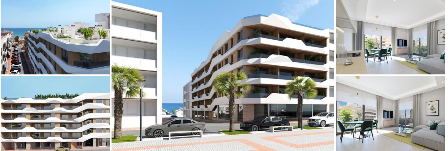
New build residential in guardamar del segura
