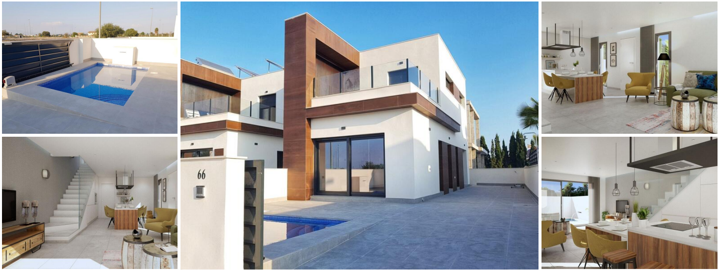
New semi-detached villas in daya nueva
