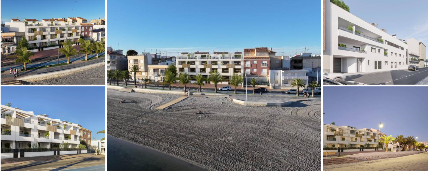
NEW BUILD FRONTLINE RESIDENTIAL IN SAN PEDRO DEL PINATAR
