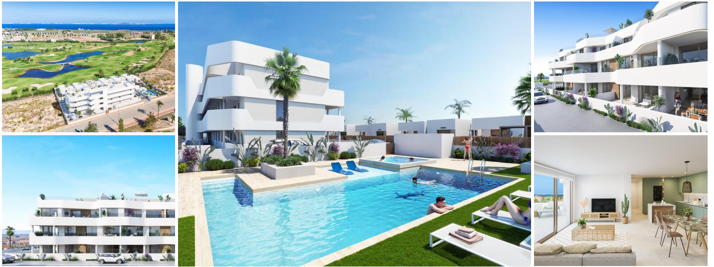
New Build Residential complex in Los Alcazares
