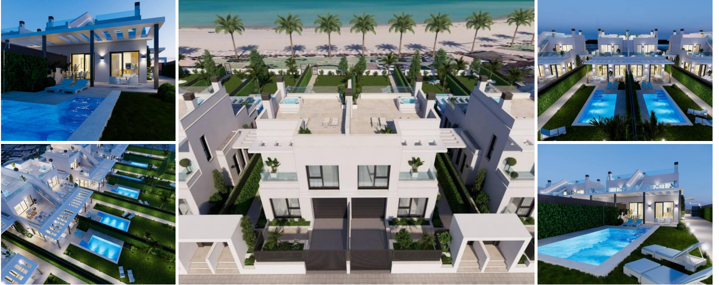
Luxury New Construction Villas on the Waterfront in Los Alcázares
