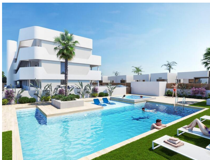
New Build Residential complex in Los Alcazares
