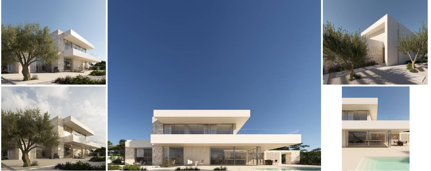
NEW BUILD VILA IN MORAIRA
