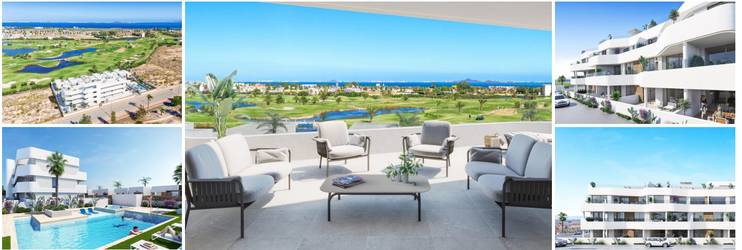
New Build Residential complex in Los Alcazares
