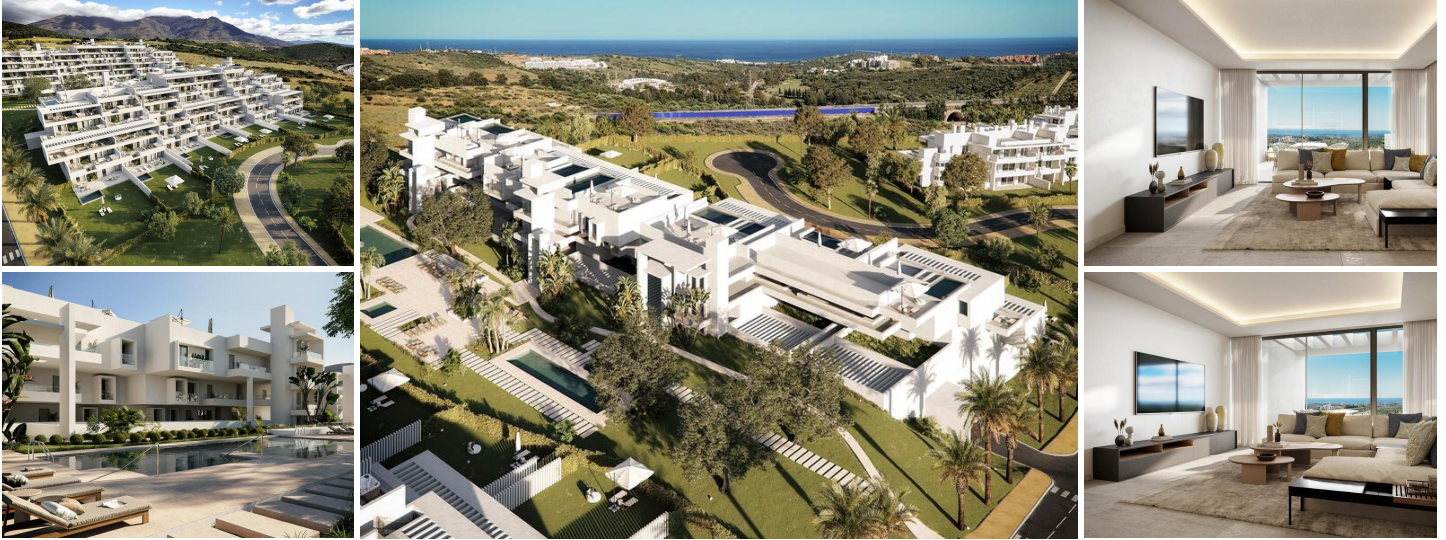
NEW BUILD RESIDENTIAL COMPLEX IN CASARES
