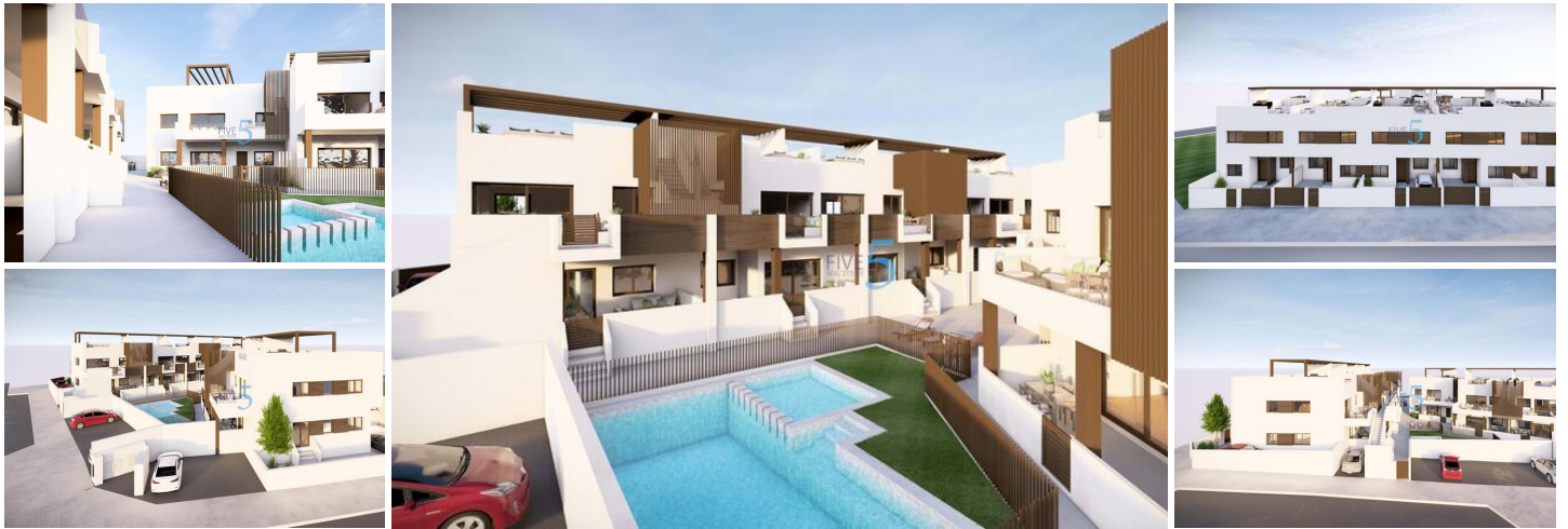
NEW BUILD RESIDENTIAL OF BUNGALOW APARTMENTS IN PILAR DE LA HORADADA
