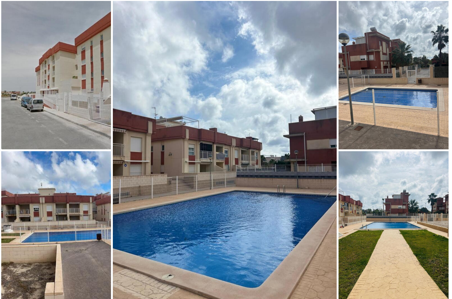
Regenerated Residential Complex in Lomas de Cabo Roig – Renovated Apartments
