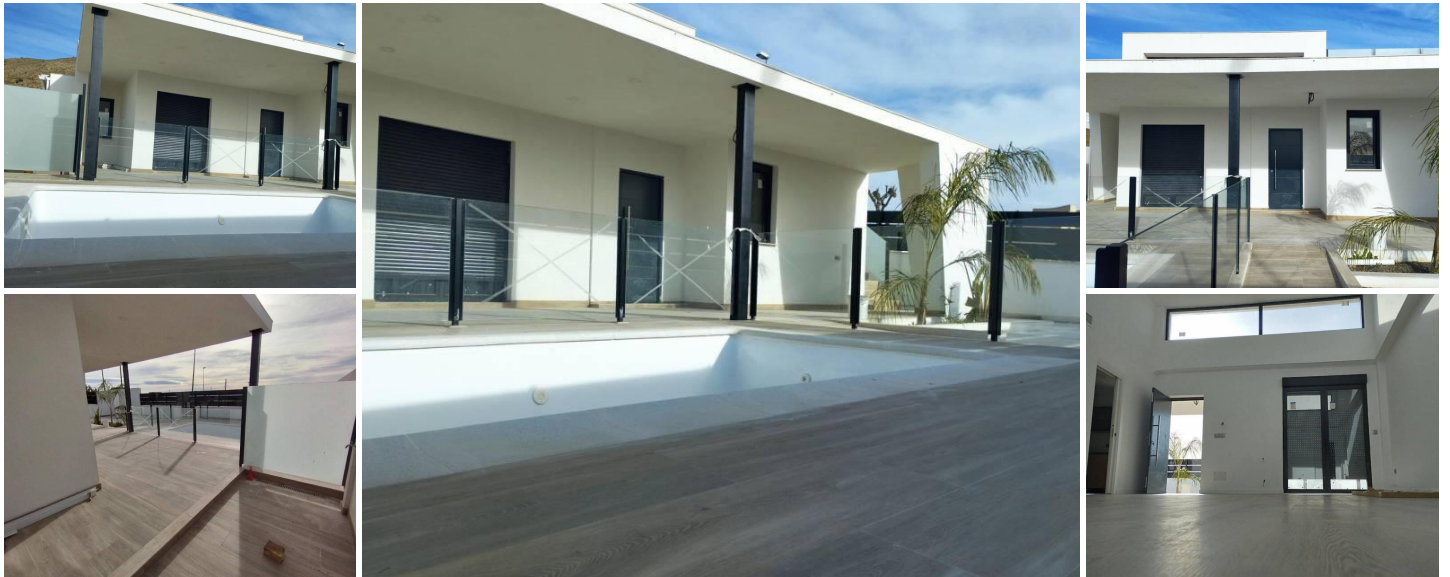
NEW BUILD VILLA IN FORTUNA
