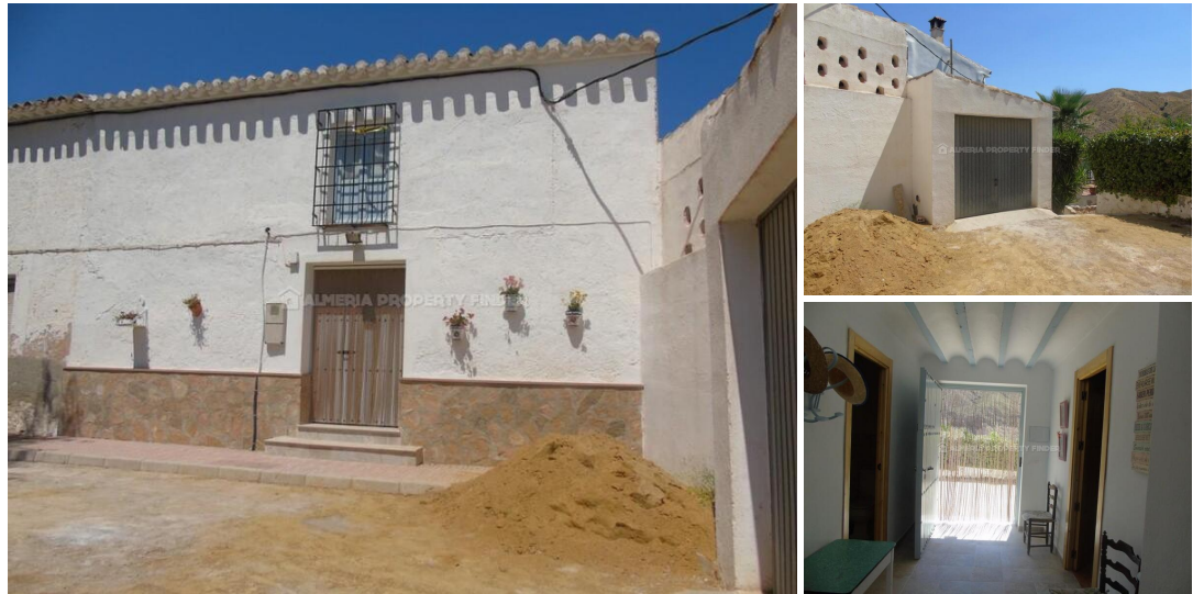
Cortijo Higuera - A country house in the Cantoria area. (Renovated)
