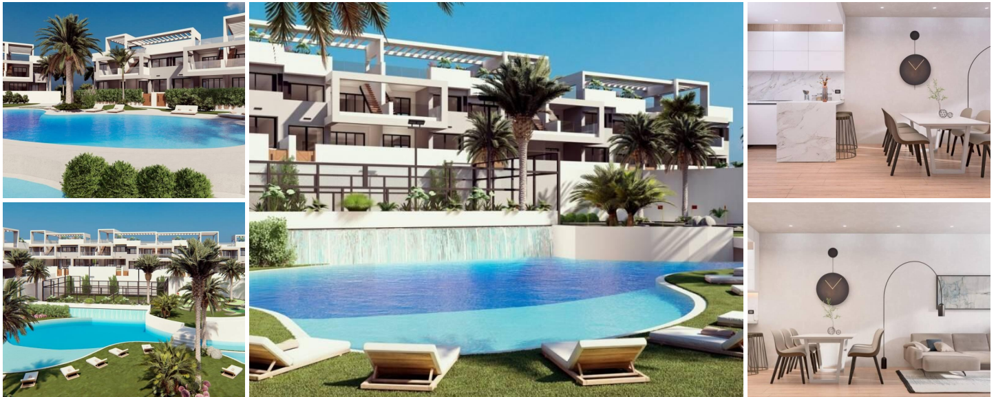
NEW BUILD RESIDENTIAL OF BUNGALOW APARTMENTS IN LOS BALCONES
