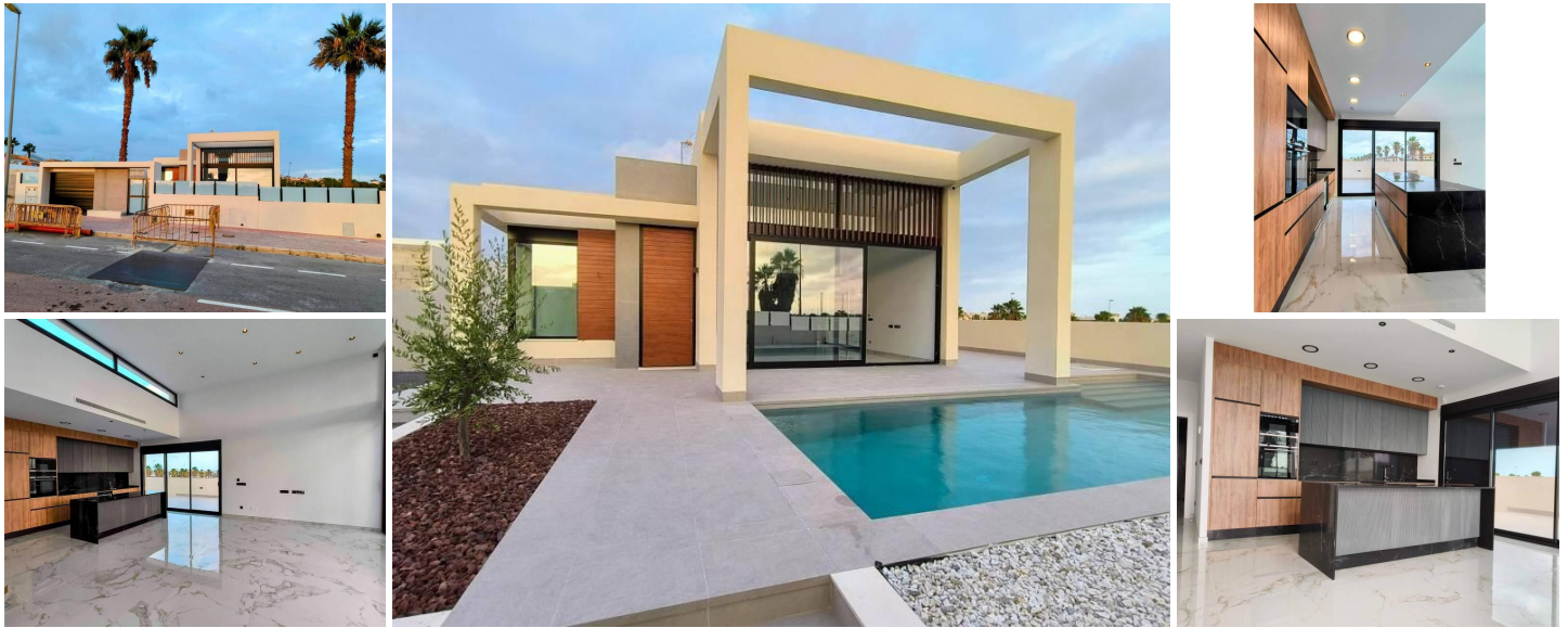
NEW BUILD VILLA IN ROJALES
