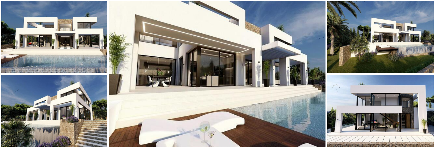
NEW BUILD VILLA IN BENNISA
