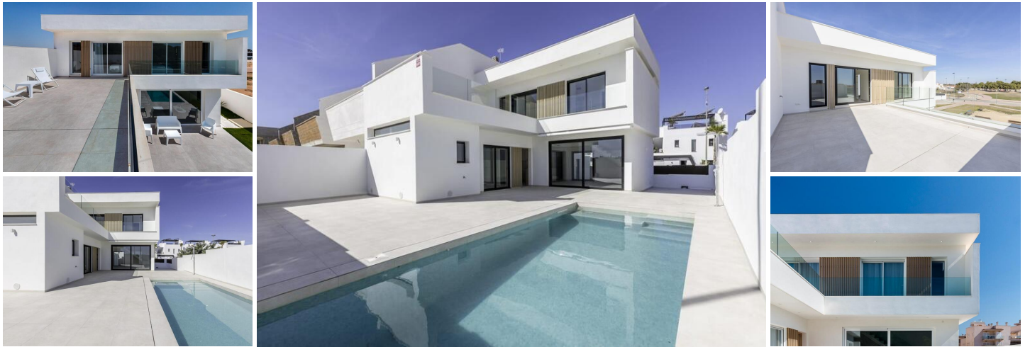
NEW BUILD SEMI-DETACHED VILLAS IN SANTIAGO DE LA RIBERA
