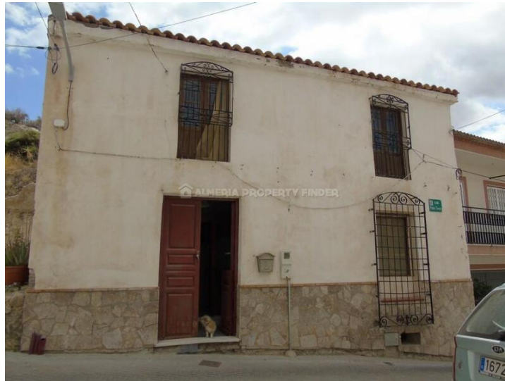
Casa Bodega - A town house in the Zurgena area. (Partially Reformed)
