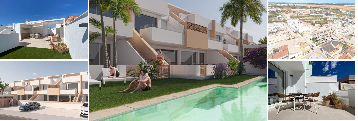
New Build Bungalows in Pilar de la Horadada Near the Beach and Town Centre
