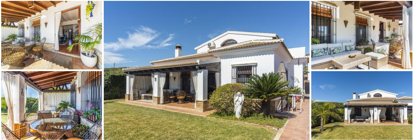
BEAUTIFUL HOUSE IN THE CARPENTER. Villamanrique of the Countess. Seville.
