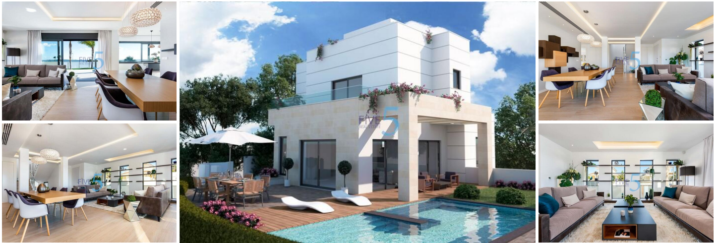
NEW BUILD VILLA IN ROJALES
