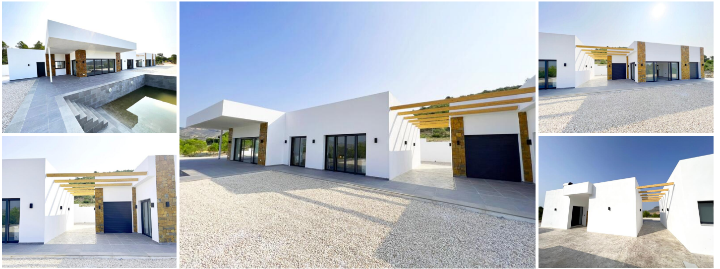
New Build Villa with Guest House in La Romana
