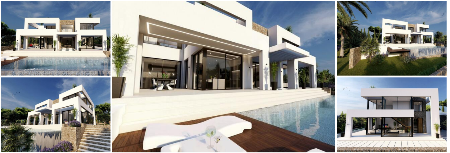
NEW BUILD VILLA IN BENNISA
