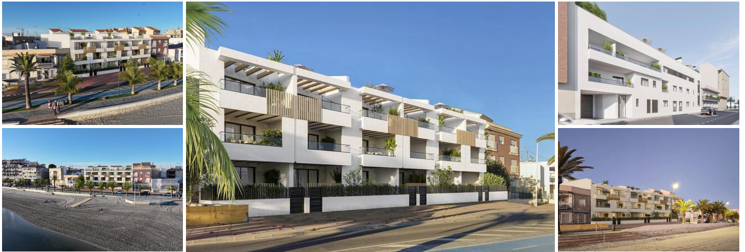
NEW BUILD FRONTLINE RESIDENTIAL IN SAN PEDRO DEL PINATAR
