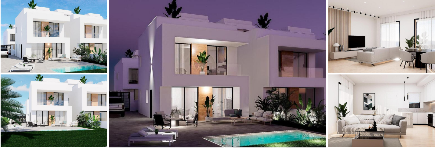
NEW BUILD VILLAS IN LA ZENIA
