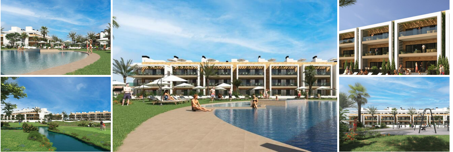
NEW BUILD RESIDENTIAL COMPLEX NEAR LA SERENA GOLF, LOS ALCAZARES
