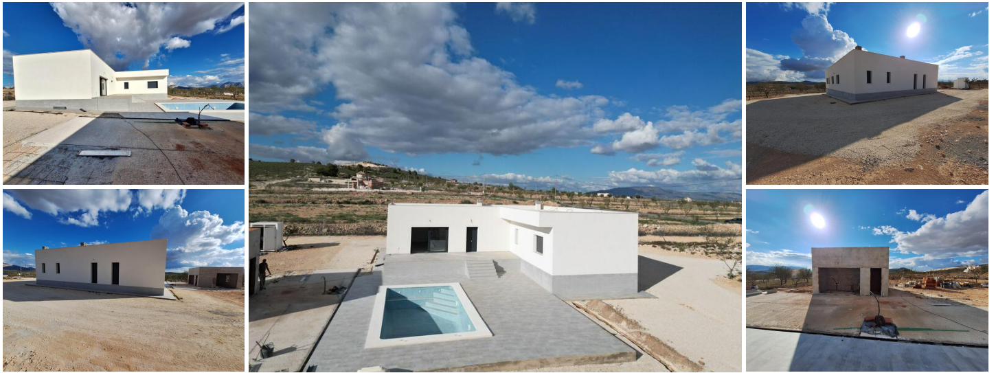
Newbuild Villa Keyready at Pinoso
