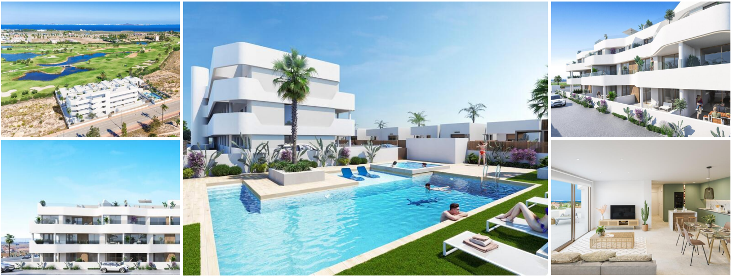
New Build Residential complex in Los Alcazares
