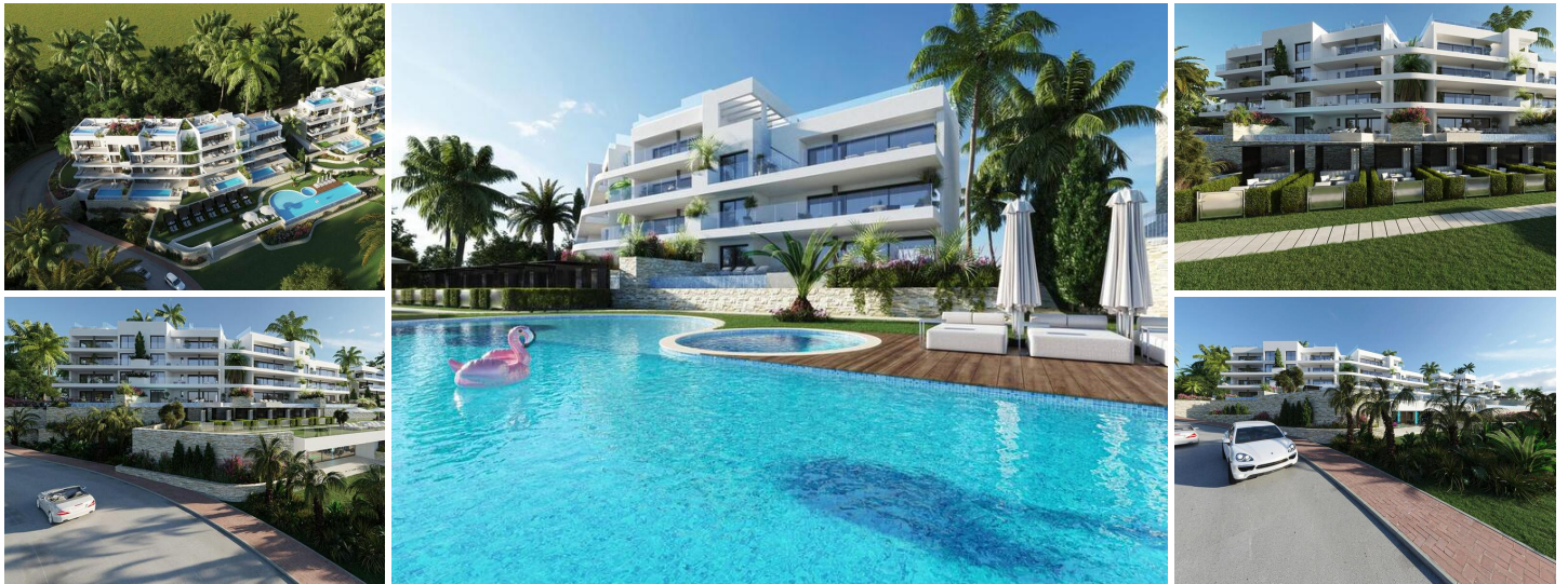
NEW BUILD RESIDENTIAL COMPLEX IN LAS COLINAS GOLF
