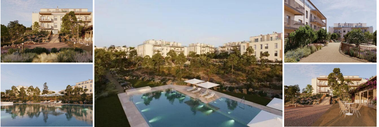
NEW BUILD RESIDENTIAL COMPLEX IN GODELLA, VALENCIA
