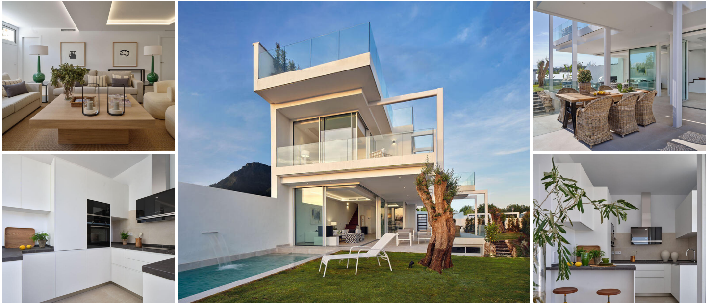
VILLA .... MARBELLA 3 Bedroom, 3 Bathrooms
