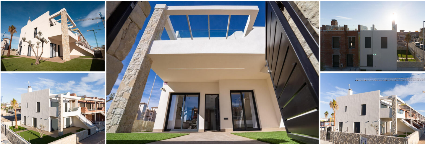
New build bungalows in Pilar de la Horadada
